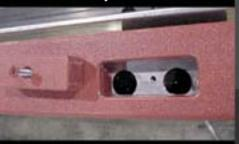
Access panel on topsill allows the glass to be easily adjusted, so it stands straight and true without any shims.
