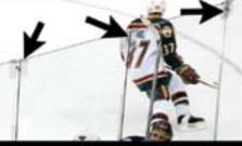
Clips allow each piece of glass to move independently upon impact, maximizing overall flexibility.
